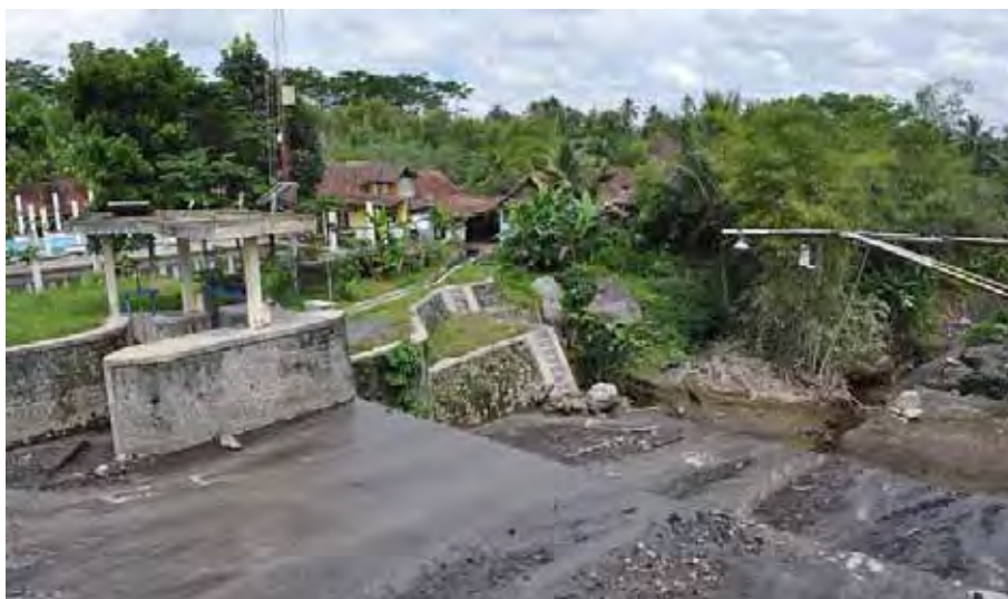
Figure 4: A sabo dam (with an outlet for irrigation)
